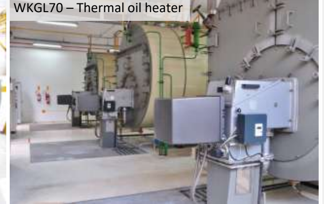
WKGL70 – Thermal oil heater
